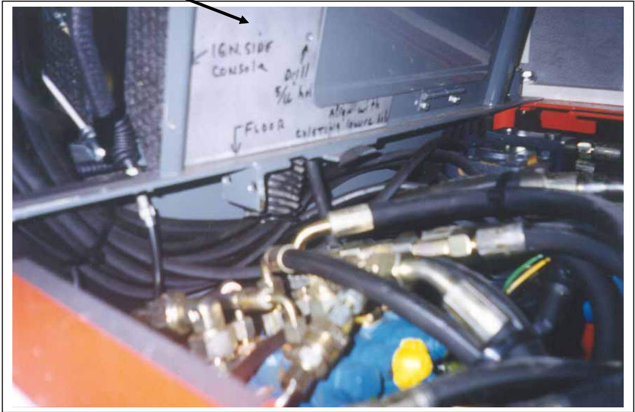
Front mounting hole template in place
